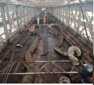
Deck planks and cross bracing removed from the bridge
